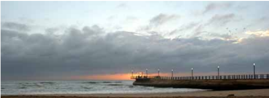
Sandile Thusi Stormwater Outfall Pier
